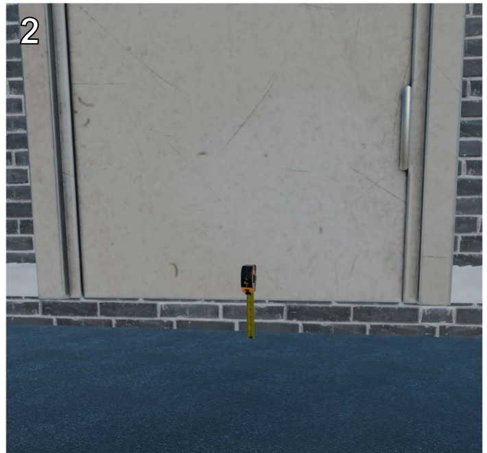
Verify height clearance is at least 2-5/8" or higher (contact salesperson for lower clearance alternatives)
