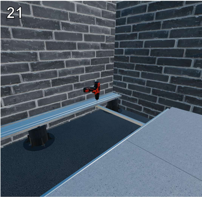
21 Using one provided screw, pre-drill and attach your final row of tracks to cross brace channel underneath the track.
